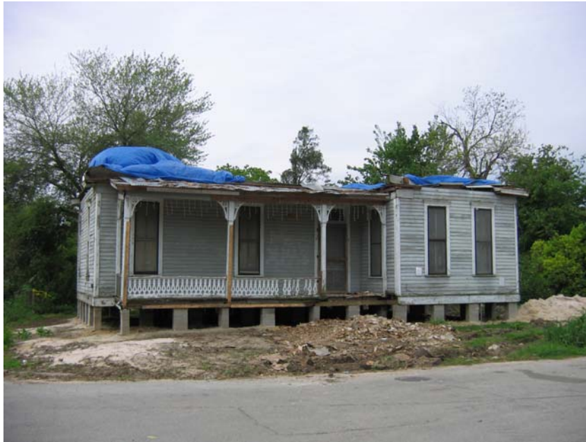
TAJAN HOUSE UNDERGOING RESTORATION AT CURRENT LOCATION
